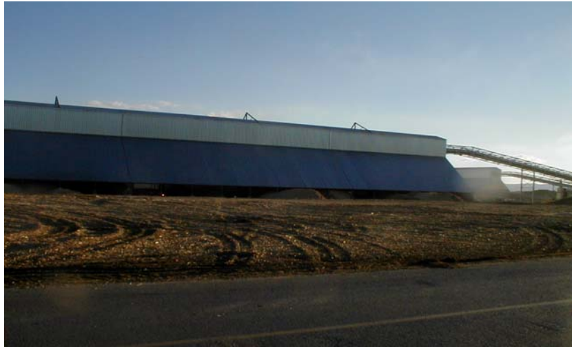
Figure 4. Tafisa's storage buildings
