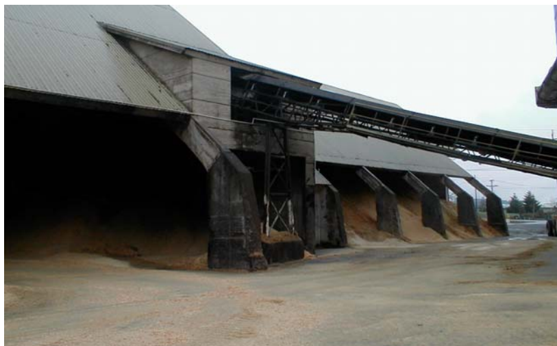
Figure 11. Duraflake's green storage building
