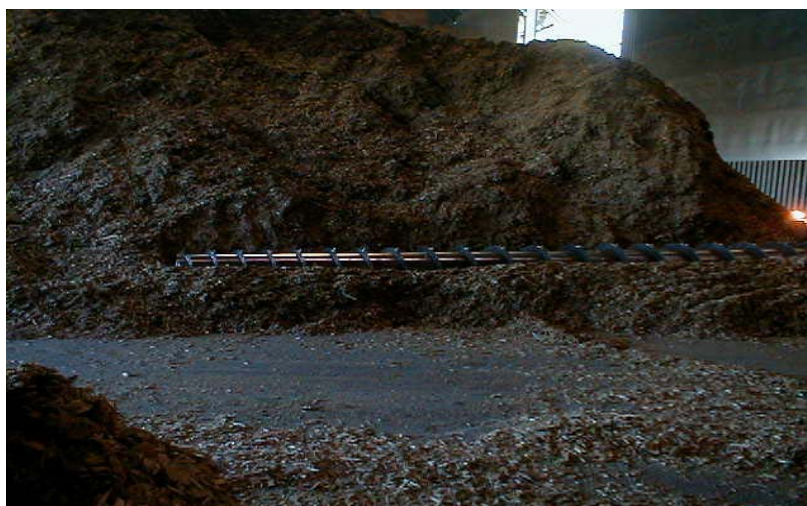
Figure 18. Tafisa's under-pile retrieval
