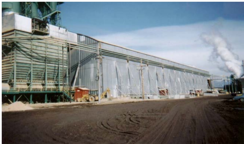
Figure 6. Plum Creek's dry storage building
